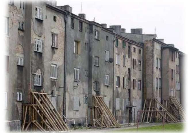
USCB mining damages
